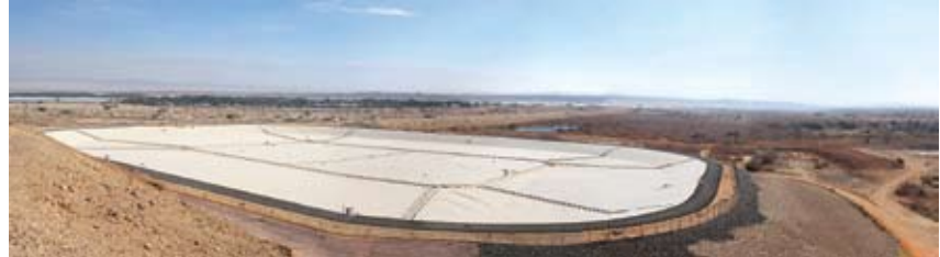
Sheizaf Reservoir covered with a Polypropylene floating cover
