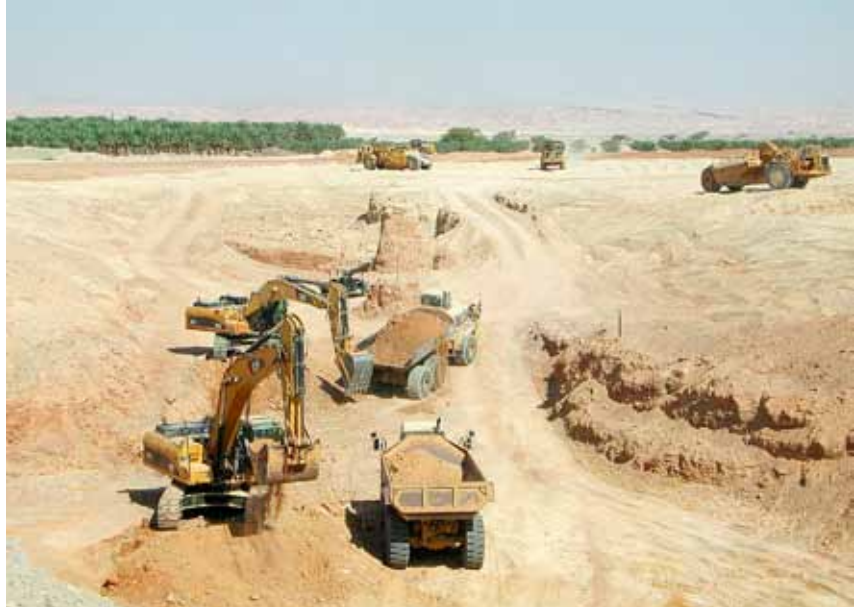
Construction of the Paran operative Reservoir. Photo by: Ami Shaham
